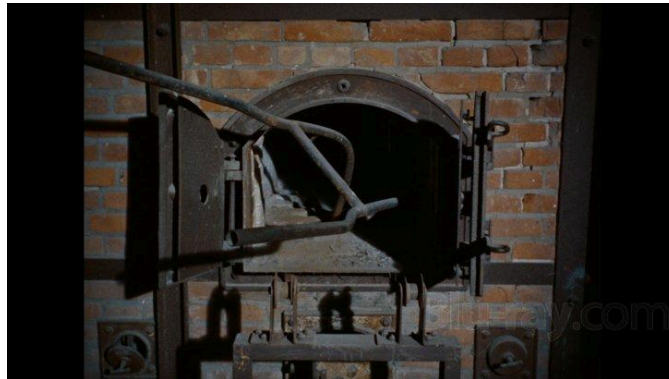
Fig 2. Incinerator that is captured in the present-day footage.
